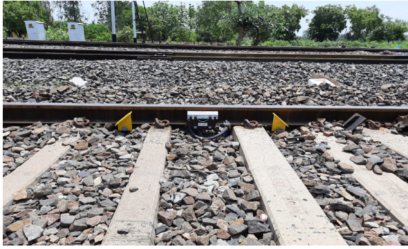
Frauscher Wheel Sensor RSR180
